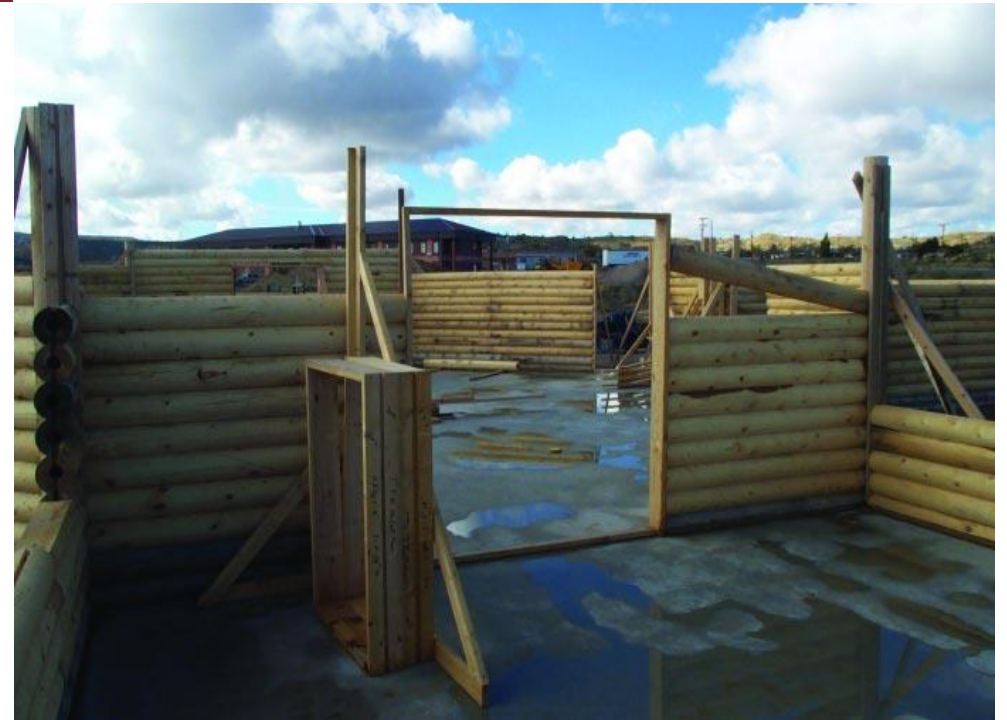
Cultural learning center under construction Crownpoint Institute of Technology (now NTU)
